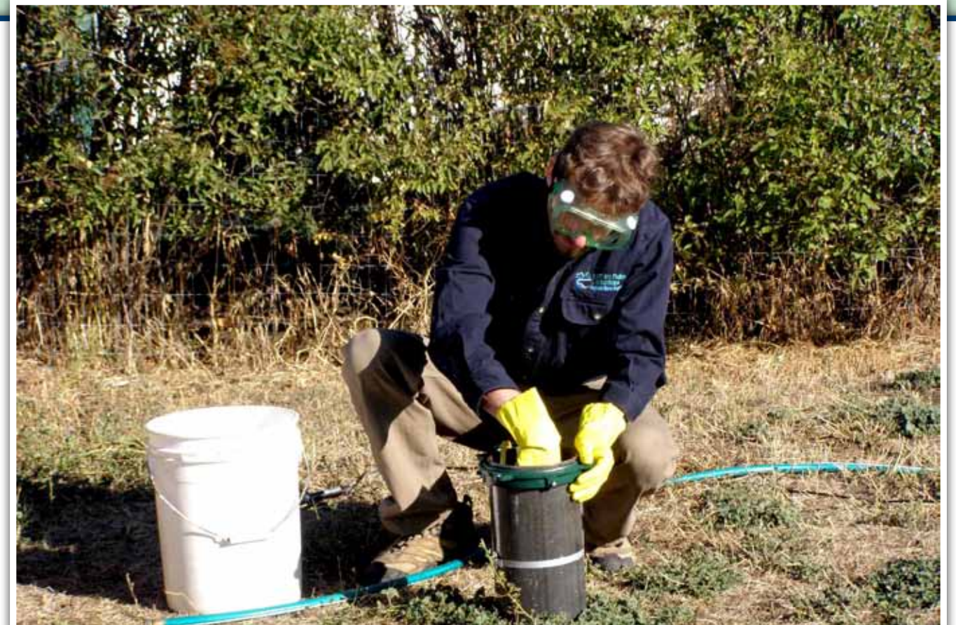
Adam Sigler (Montana State University) demonstrates the process of shock chlorinating a well for the "Taking Care of yOur Ground Water" DVD. Courtesy of Suzanna Carrithers Soileau, formerly Montana State University; currently USGS-Bozeman, Montana
